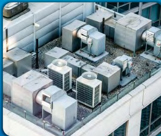
Commercial Combustion Water/Space/Heating/ Cooking/Others
