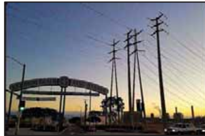
Remove utility visual blight
